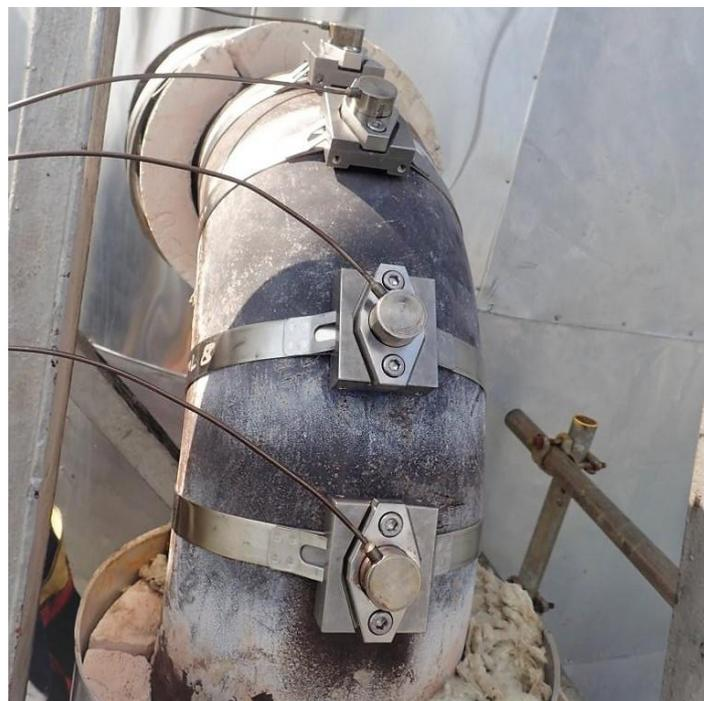
Figure 3: A photograph of four high-temperature HotSense™ ultrasonic wall-thickness monitoring transducers with integrated calibration block, installed on a refinery crude distillation unit (CDU), 8” diameter carbon steel outlet pipe operating at 350 °C continuously, under insulation (removed for photo) (Photos © Ionix Advanced Technologies 2020).
