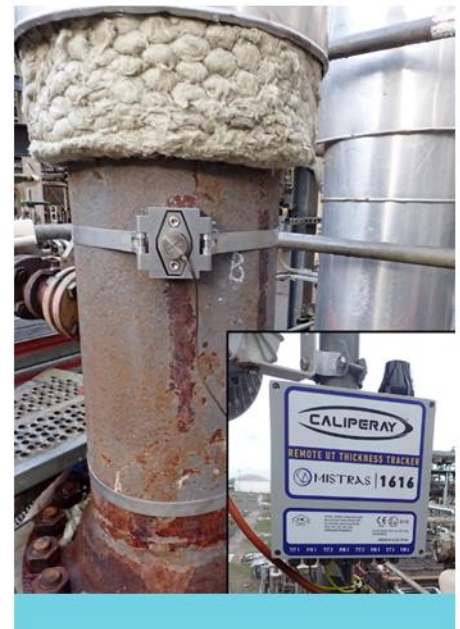
Figure 1: HotSense™ and CALIPERAY installation
