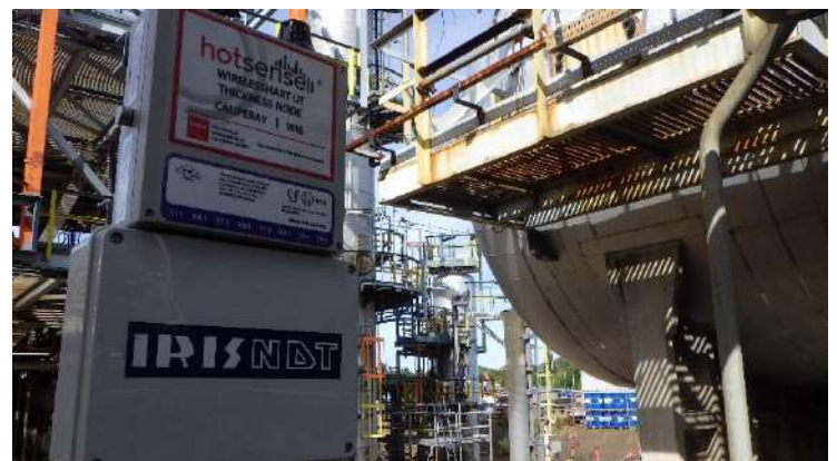
HotSense CALIPERAY Wireless UT Monitoring System
