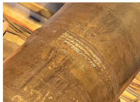
Figure 2: Photograph of the pipe weld inspected at 200 °C.
