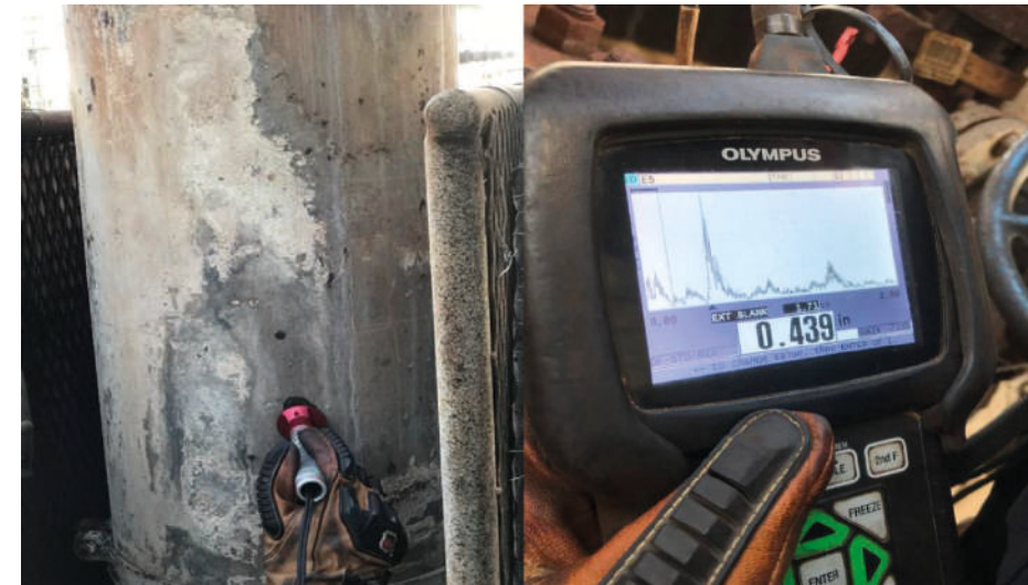
Fig. 1 (Left) Ionix HS582i probe in use at US Oil Refinery by a Inspector. Pipe temperature readings at time of this inspection were 582°F (305°C). (Right) The thickness measurements were able to be repeated several times with minimal cool down periods.
